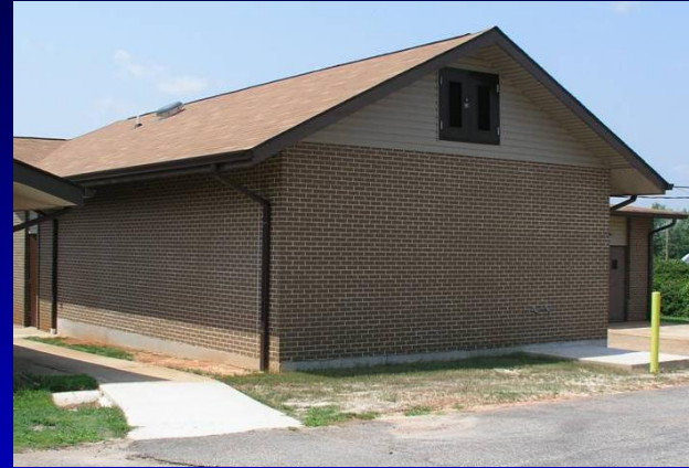
New addition prior to cold room
